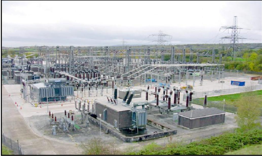
**Figure 8.4:** Air Insulated Substation (Source: <http://www.foxitsoftware.com>)
