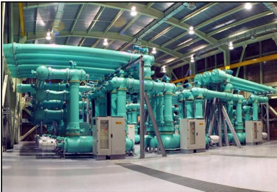
**Figure 8.3:** Gas insulated Substation (Source: <http://kiran111.hubpages.com/hub/Gas-Insulated-Substation> 24-06-2013)
